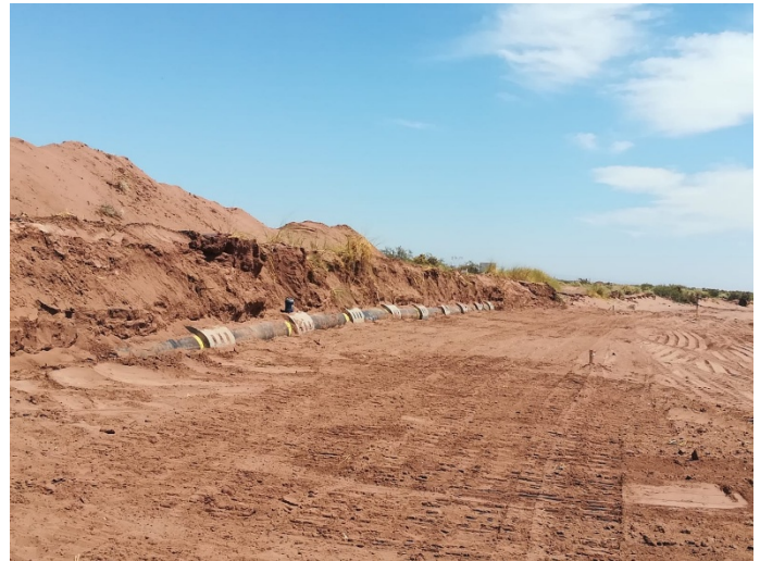
FIGURE 25: BOLT-ON WEIGHTS PLACED ON THE EXPOSED SEGMENTS
