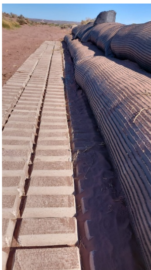
FIGURE 27: BANK PROTECTION WITH GEOTUBES
