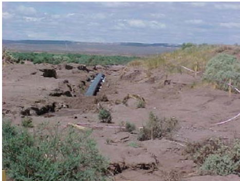
FIGURE 18: PIPELINE EXPOSED AT THE EDGE OF FLOODPLAIN AFTER THE 2004 FLOOD
