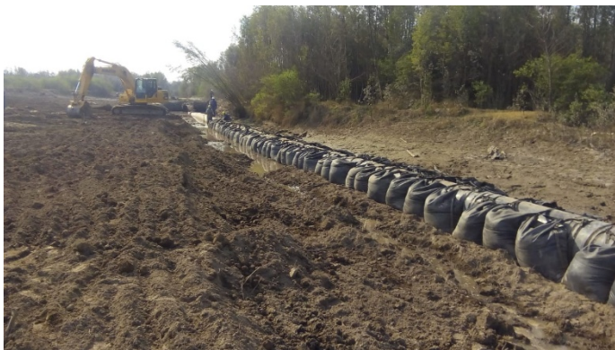
FIGURE 10: SOIL FILLED BAG WEIGHTS PLACED FOR PRELIMINARY REMEDIATION
