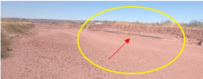
FIGURE 23: EXPOSED PIPELINE ALONG LEFT BANK
