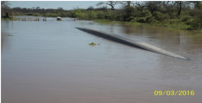
FIGURE 8: BUOYANCY OF 30" LINE AFTER YEAR 2016 FLOODING
