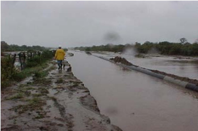
FIGURE 7: BUOYANCY OF 24" LINE AFTER YEAR 2000 FLOODING
