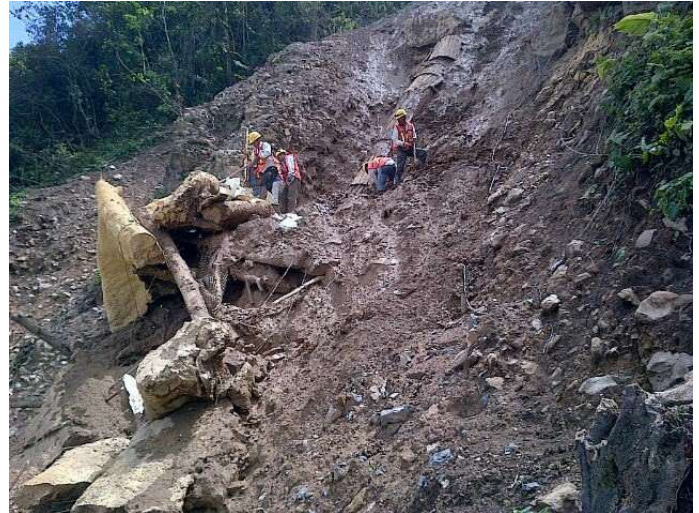
FIGURE 9: TRENCH BREAKERS FAILURE. AFTER COLLAPSE, THE PIPE WAS EXPOSED AND DAMAGED.
