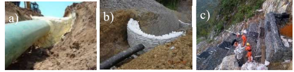
FIGURE 4: TRENCH BREAKER MATERIALS. FOAM (A), SANDBAG (B), AND GABIONS (C).
