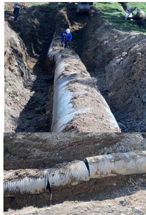
FIGURE 13: DISPLACEMENT AND EXTERNAL CASING FRACTURE OBSERVED AT THE UPSTREAM FLANK OF THE MOVEMENT (SOURCE: CENIT)
