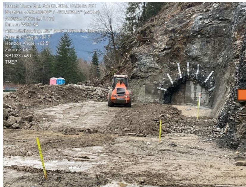
Cut Face Mitigation at a tunnel portal
