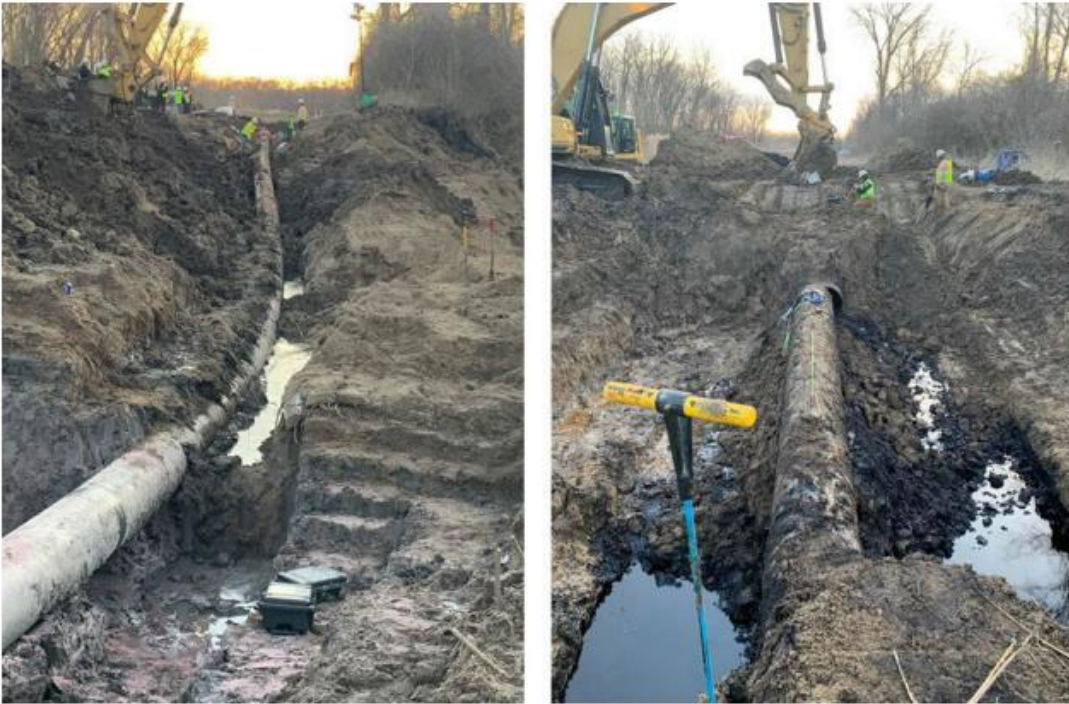
Figure 1.1: Failed Girth Weld During Excavation
