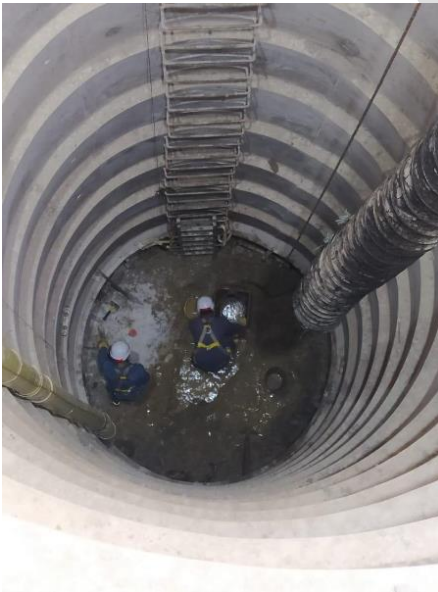
FIGURE 4. Horizontal drain collection chamber for piezometric level reduction. Source: Specialized web site
