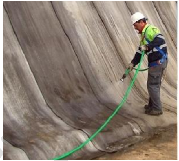
FIGURE 5. Concrete mats for slope protection. Source: Specialized web site
