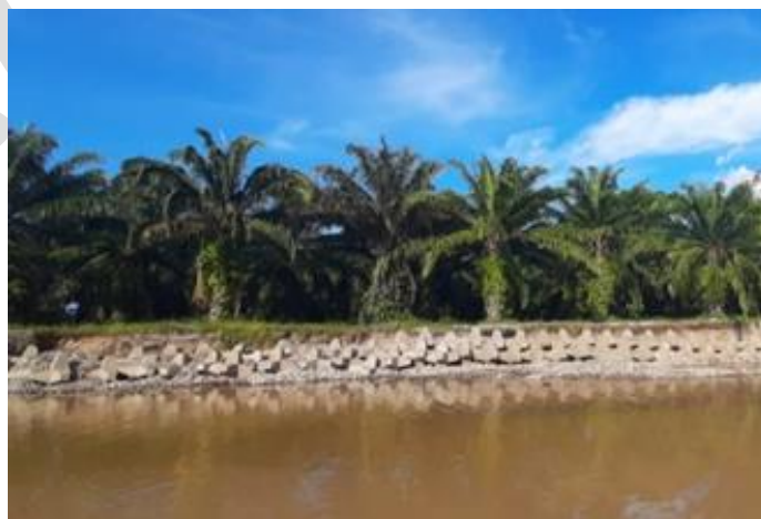
FIGURE 2. Riverbank defense with concrete blocks. Source: Specialized web site.
