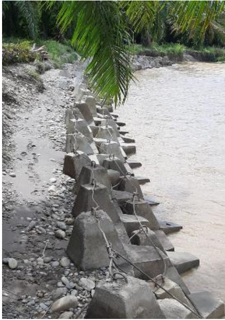
FIGURE 3. Riverbank defense with concrete dice Source: Specialized web site
