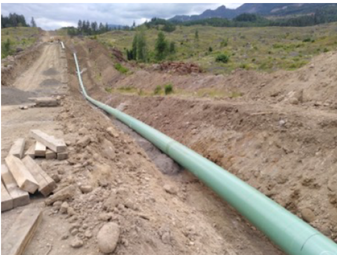
FIGURE 4: PIPELINE LOWERED INTO THE EXCAVATED TRENCH.
