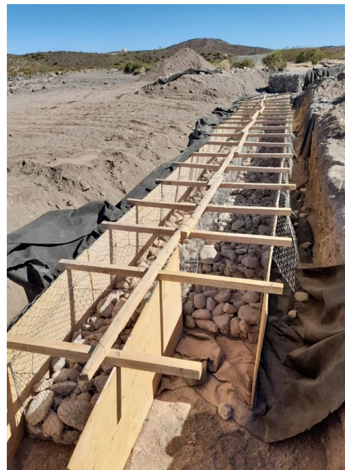
Image 16 – Construction of foot protections to prevent undermining - Source: Author of the paper
