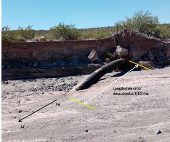
Image 4 – Exposed pipeline – Source: Author of the paper
