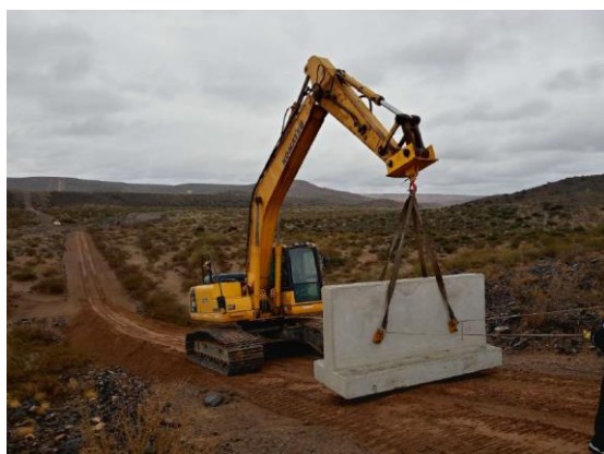
Image 15 – Equipment moving a sleeper – Source: Author of the paper
