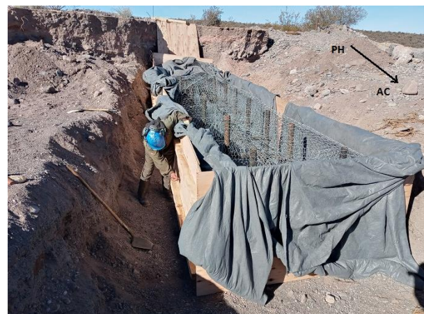
Image 12 – Construction of temporary work with gabions and reinforcement tubing – Source: Author of the paper
