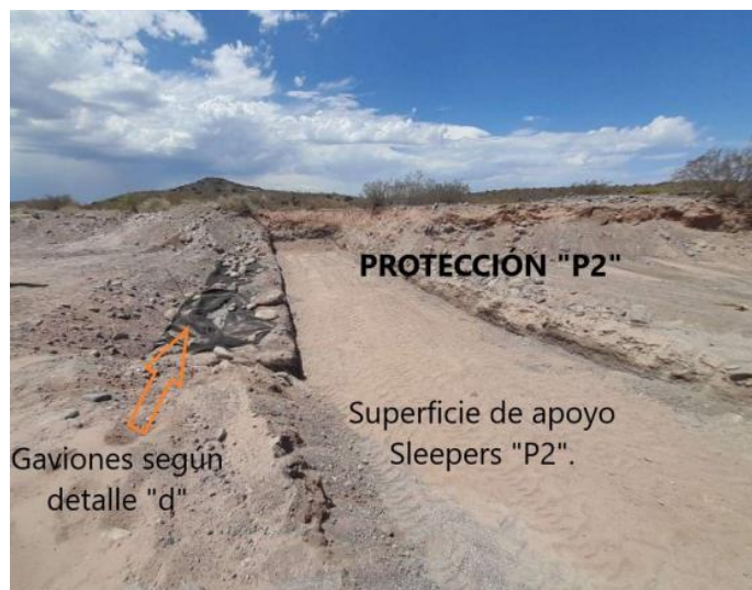
Image 17 – Preparation of inclined surface for the placement of sleepers - Source: Author of the paper
