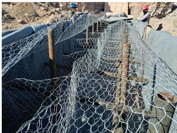
Image 11 – Construction of temporary work with gabions and reinforcement tubing – Source: Author of the paper
