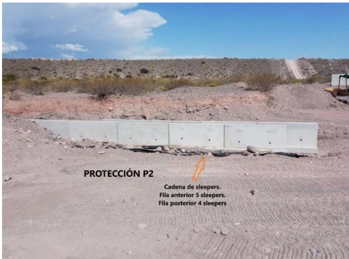
Image 18 – Sleepers in final position - Source: Author of the paper
