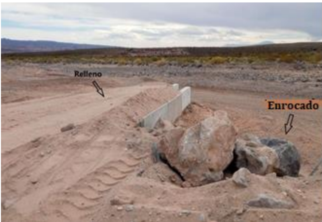
Image 23 – Materialization of erosion protection rocks - Source: Author of the paper
