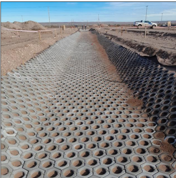
FIGURE 20: SOUTH CHANNEL SECTION IN HR60 BLOCK
