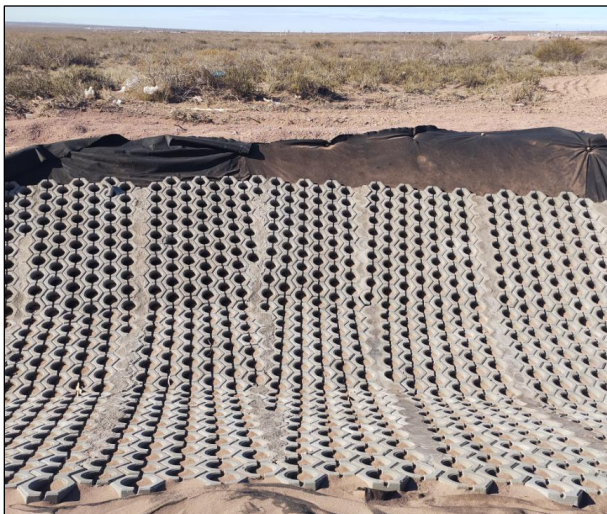
FIGURE 24: DETAIL OF JOINTS IN CURVED HR60 BLOCK
