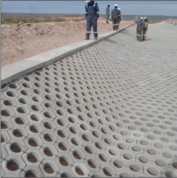
FIGURE 19: NORTH CHANNEL SECTION IN HR80 BLOCK
