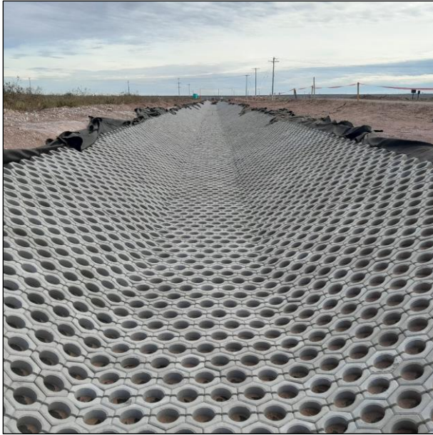
FIGURE 23: CHANNEL IN HR60 BLOCK
