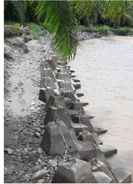
FIGURE 3. Riverine defense with concrete blocks. Source: Internet (2020).
