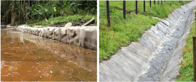
FIGURE 6. Concrete coating for water control. Source: Internet (2020).
