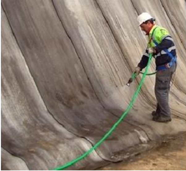
FIGURE 5. Concrete coating for slope protection. Source: Internet (2020).
