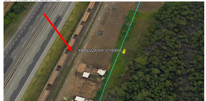
FIGURE 24: GOOGLE EARTH IMAGE FROM JUNE 2018, DISPLAYING THE PRESENCE OF TWO ADJACENT RAILWAY LINES.
