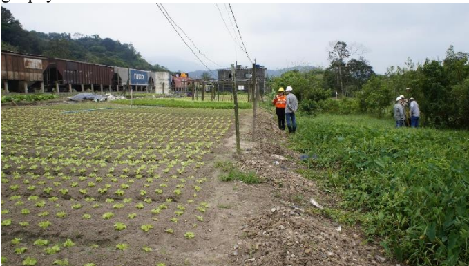
FIGURE 2: AT-GRADE PHOTOGRAPH DEPICTING THE SITE WHERE THE ARC-SHAPED DEFORMATION IMPACTED THE GAS PIPELINE.
