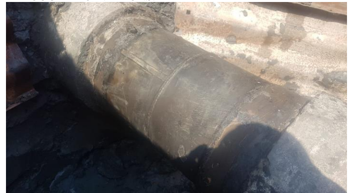
FIGURE 32: PHOTOGRAPH OF THE EXCAVATED PIPELINE JOINT FOR SUPPLEMENTARY STRESS ANALYSIS INSPECTIONS.
