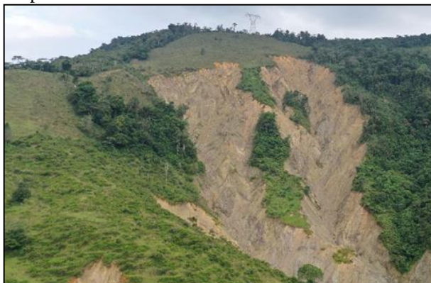
FIGURE 13: PROGRESSION OF SLOPE DEGRADATION NEAR A POWER TOWER
