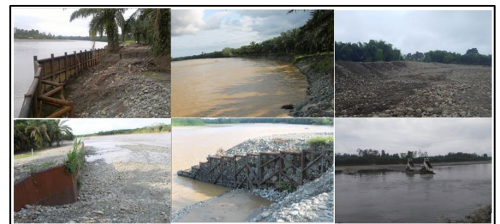
Figure 13: Sequence of implemented erosion control works.
