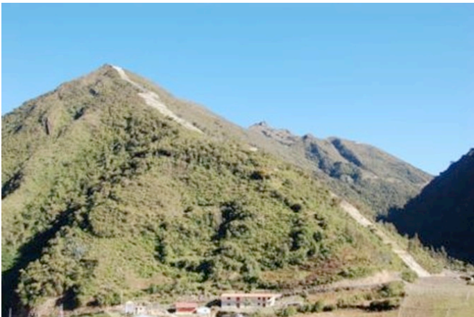
FIGURE 2: PIPELINE ROW NEAR CHIQUINTIRCA, SIERRA REGION
