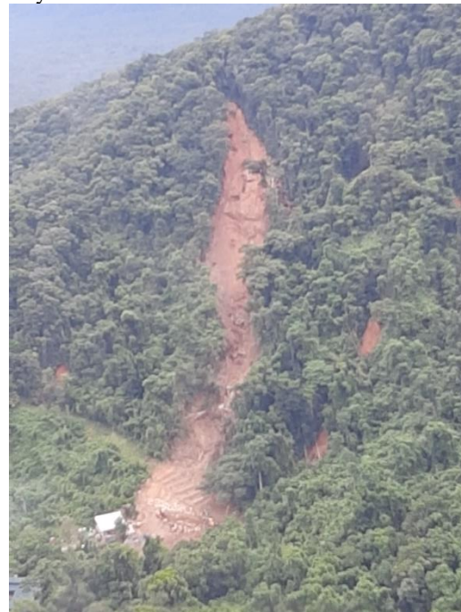
Figure 5: km 41+100 - Deposited mass on the right-of-way
