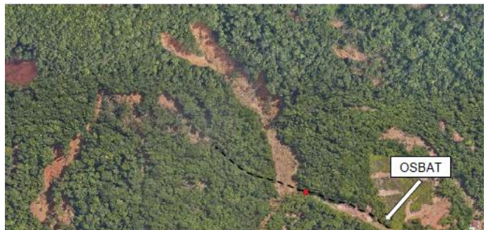
Figure 2: Aerial view showing large landslides. (3)
