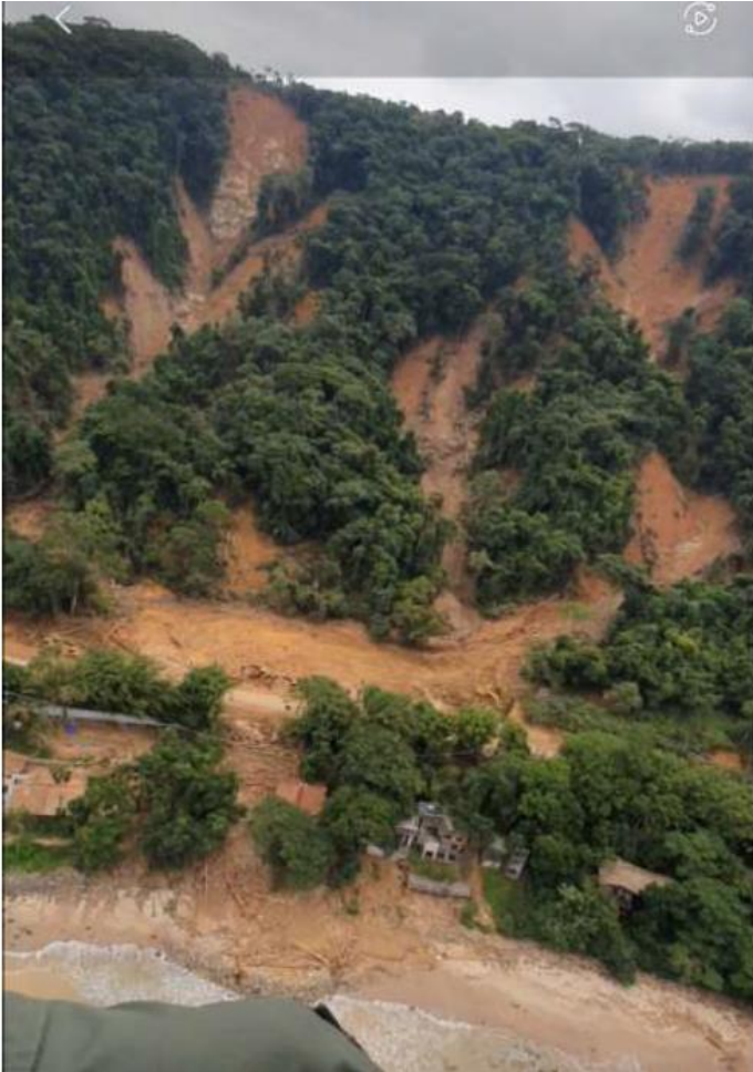
Figure 3: km 37+000 - Three debris flows crossing the right-of-way and the road reaching the shore. (4)
