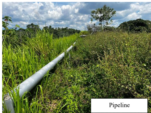
FIGURE 4 ABOVE: THE GABION WALL IS OBSERVED WITH A DEFORMATION IN ITS HEAD. BELOW: THE EXISTING FLOW LINE THAT WAS INSTALLED AT THE TOP PART OF THE WALL.
