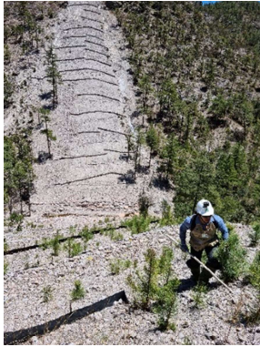
FIGURE 16: PRESENCE OF STREAM CUTTERS IN RIGHT OF WAY
