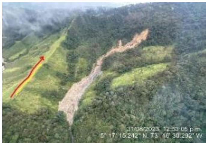
FIGURE 7: Flow of soils over a ravine. The mass was dammed for a large rock under a bridge. Source: OCENSA, aerial patrol.
