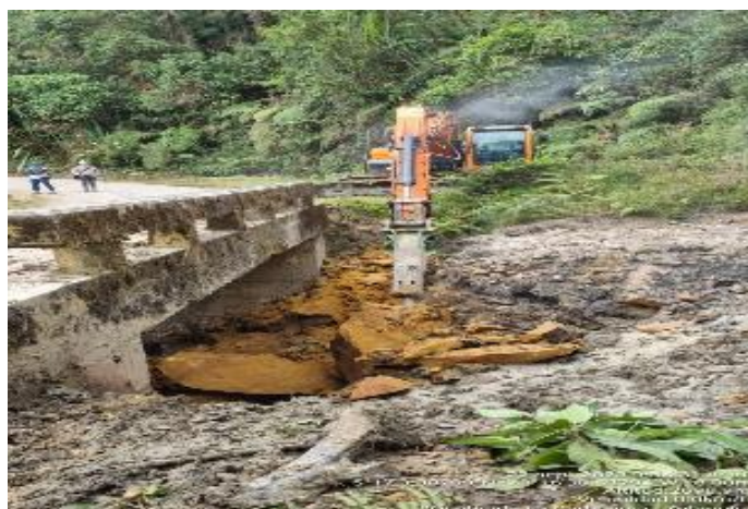
FIGURE 8: Demolishing of the rock under the bridge. Source: OCENSA
